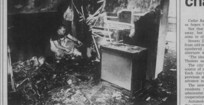
Oelwein Fire Chief Wallace Rundle indicates the place where a fire started early Monday in an upstairs apartment on Lincoln Drive. The fire in the apartment of Marsha Corbin started behind a stereo from a short in an extension cord. The fire gutted the residence and caused an estimated $12,000 in damage. Marsha Corbin, who lived alone, was the occupant of the downstairs apartment was home when the fire broke out. Rundle said. A neighbor discovered the blaze and summoned firefighters about 6:30 a.m.
